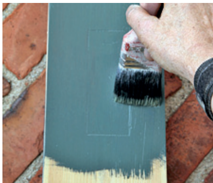
Spread the paint out well in several directions. Finish off following the grain of the wood.
