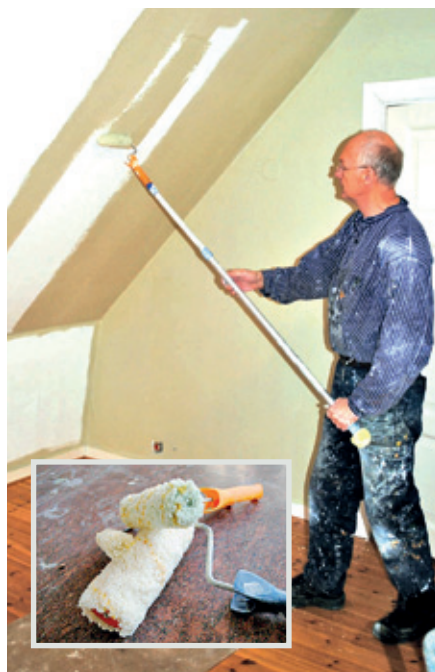
Painting papered walls with a roller.
