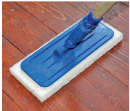
Linseed Oil Wax is applied lightly with a rough sponge, e.g. Scotch Brite.
