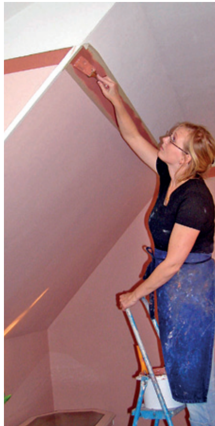
Paint Linus using a Perlon roller or a brush.
